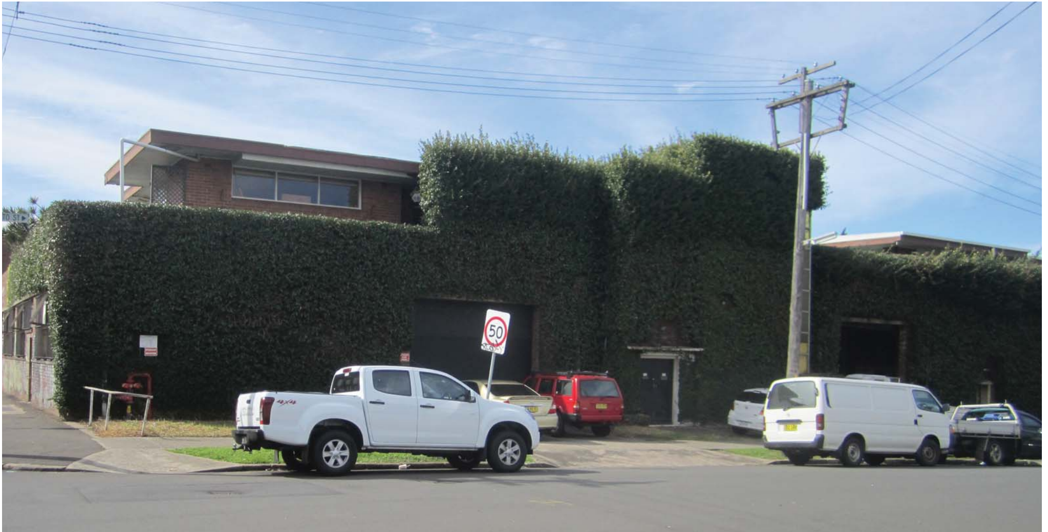
Alberto Street frontage
