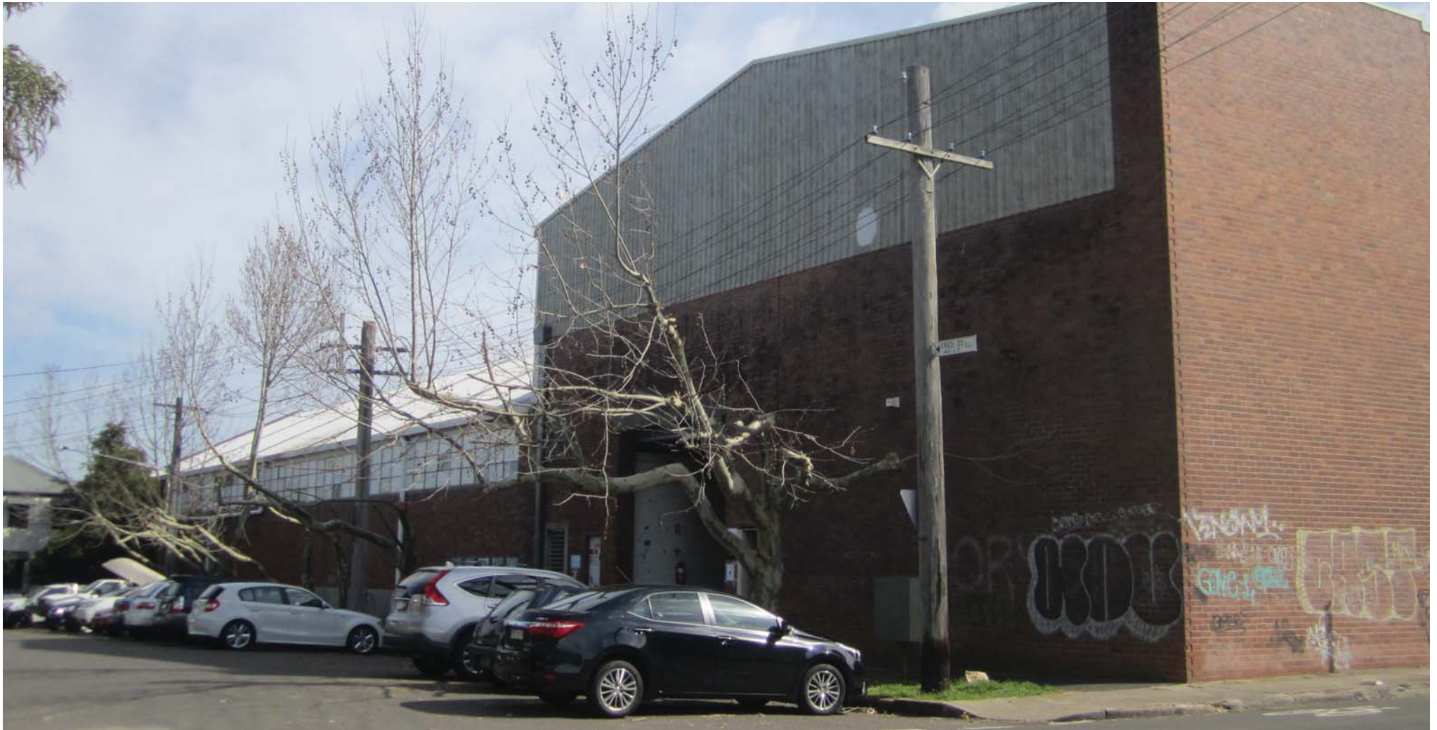
Fred Street frontage
